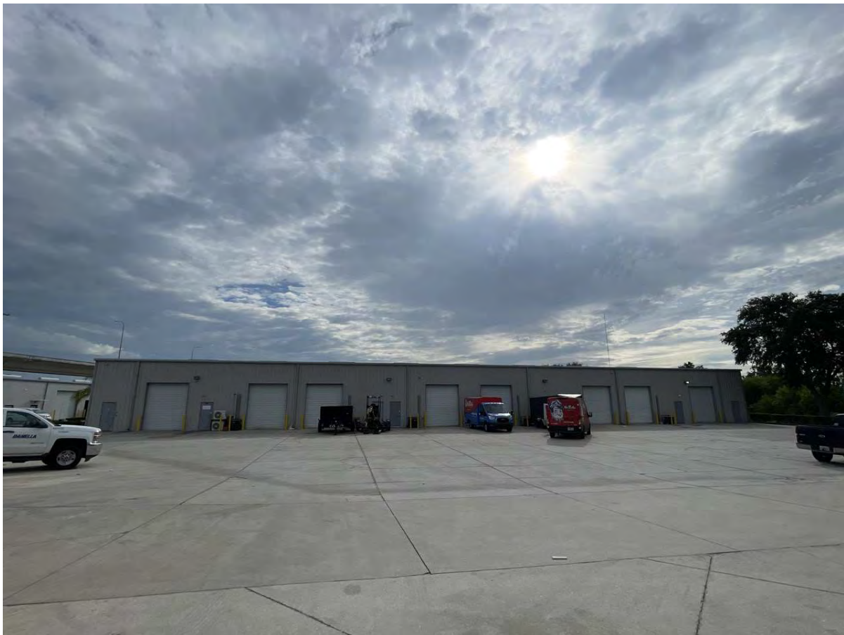
Site 044 – Zimek Technologies LLC, 251 78 th St; View of building frontage and rear loading bays.
